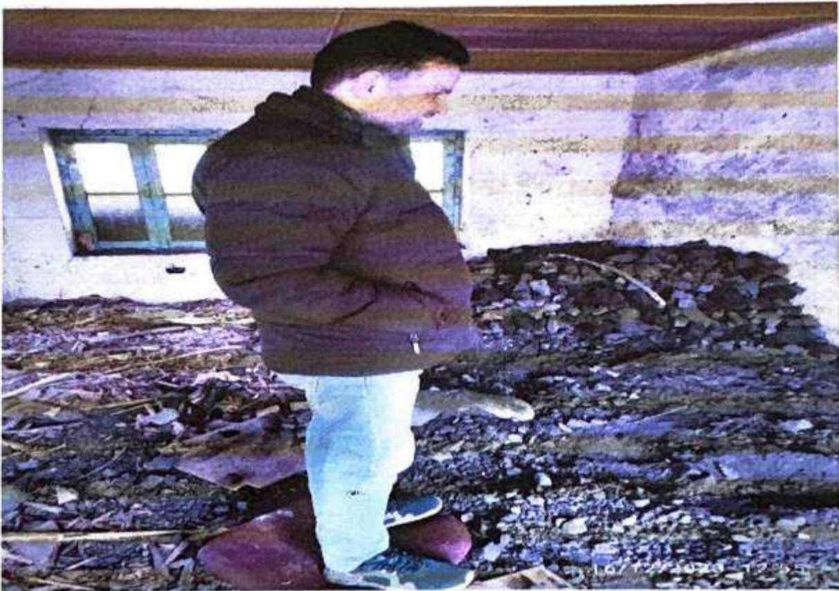
Fig.5. College shed used to store hard Coal
